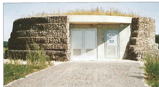
Station de pompage Oberen-Erlen
